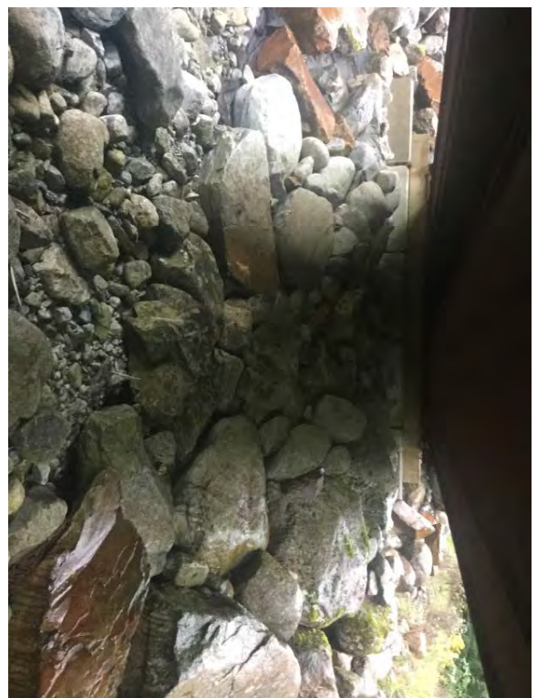
Left Bank Abutment when facing downstream
