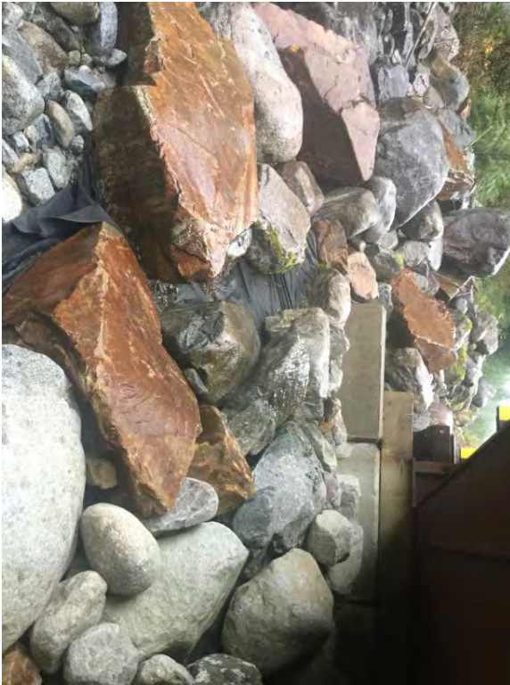
Left Bank Abutment when facing downstream
