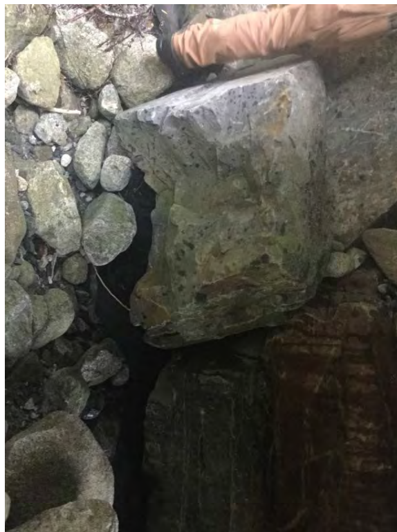
Right Bank Abutment when facing downstream
